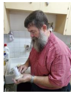
Kitchen sink repair
